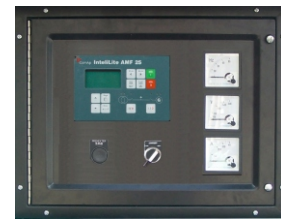
The controller made in Turkey Comap genset controller
